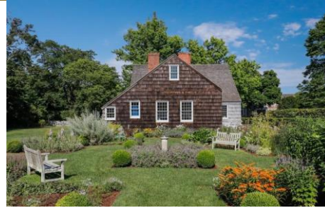
Halsey House 249 South Main Street, Southampton
